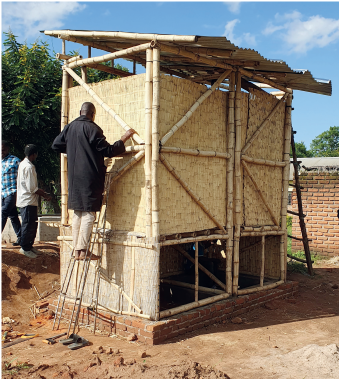
Figure 19: Construction of Dry Toilets Pilot / Source: Gerd Runge 2023
