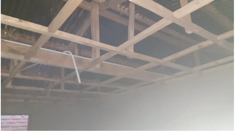
Figure 13: Ceiling structure on hostel houses /Source: Chingalire 2022
