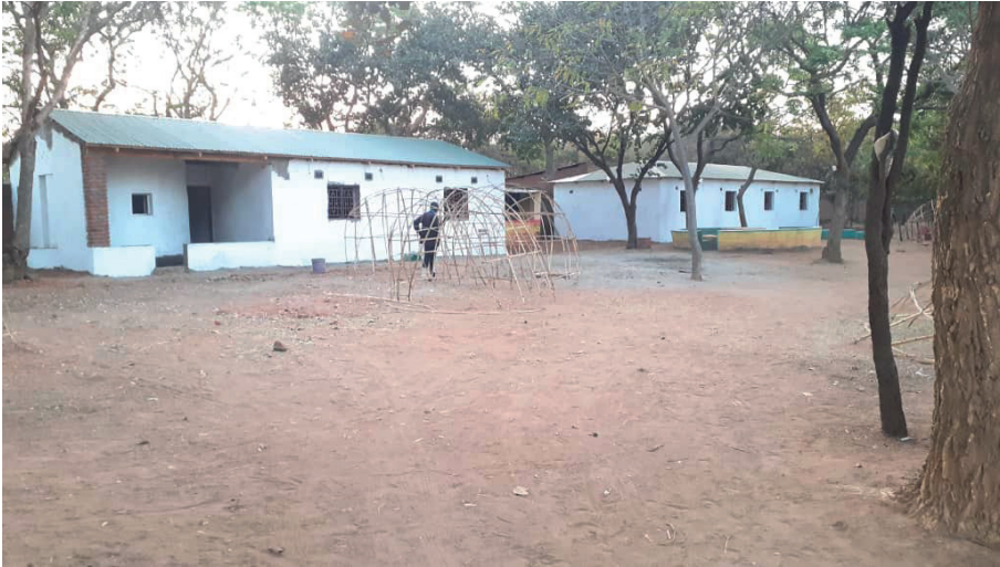
Figure 10: Finalised construction of hostel houses /Source: Chingalire 2022
